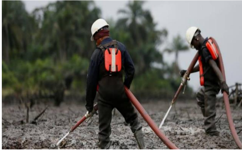
Figure 1: An Oil Spill Response Using High Pressure Water Technique.
